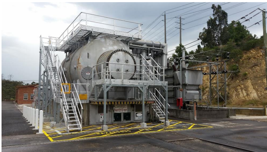
Figure 3: a synchronous compensator at Templestowe substation, Melbourne Victoria, Australia (source: Wikimedia Commons)
